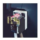
Depending on the servomotor fitted to the burner, a three-pole potentiometer (1000  $\Omega$ ) can be installed to check the position of the servomotor.
