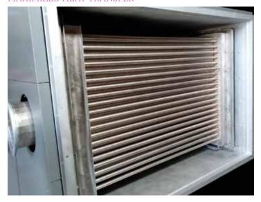
The tube bank of the indirect fired – ITAS Horizontal flow hot air generator offers a large surface for improved heat-transfer and maximum efficiency.
